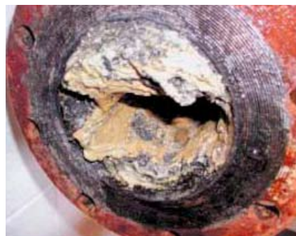
A pipe clogged with hardened grease
